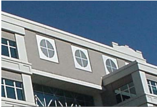
Figure 8a: 151 South 4 th Street
